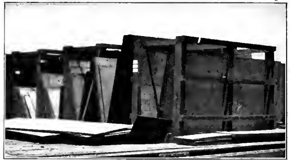
Rack for Storing Boiler Plate
